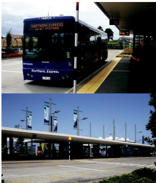
Figure 3 Northern Express Bus Station (Photos taken by Authors)
